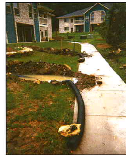
Soil slope and wetness need to be evaluated before basement construction.
