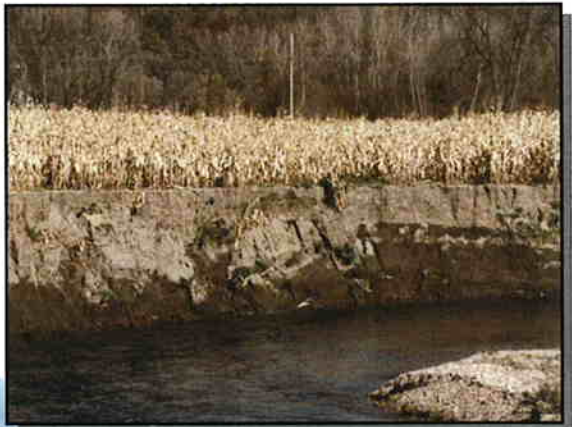
Erosion occurs when the natural vegetative buffer is removed.
