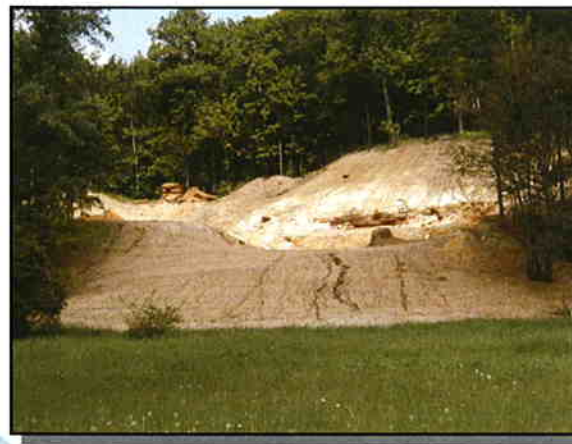
Bluffs are highly susceptible to soil erosion.
