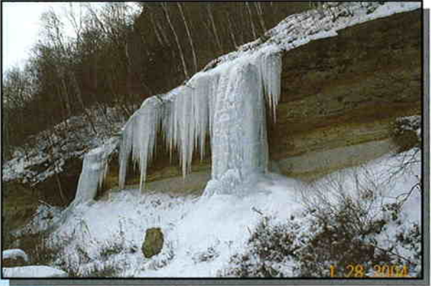
Disturbed ground has exposed groundwater flow over the St. Lawrence Edge
