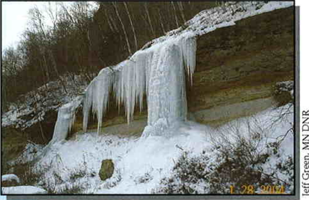
Disturbed ground has exposed groundwater flow over the St. Lawrence Edge
